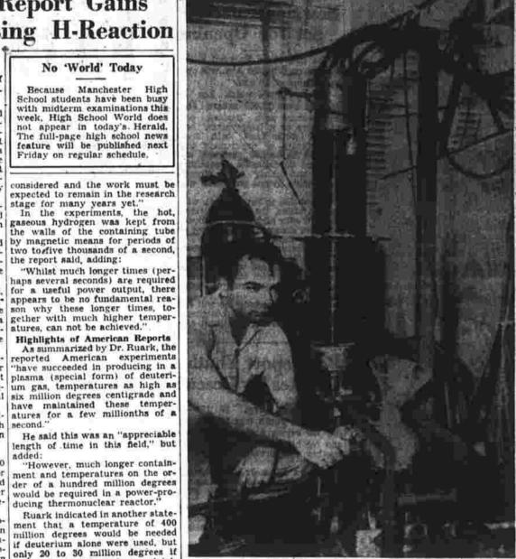
Technician Lew Burkhardt adjusts a valve alongside the coilwrapped upright tube which is the heart of the hydrogen fusion device at the Atomic Energy Commission's Los Alamos, N. M., laboratory. The tube encases a smaller container of deuterium or heavy hydrogen gas. The small funnel feeds liquid nitrogen at 273 degrees below zero into a tank which acts as a filter for a pump evacuating all but heavy hydrogen gases
